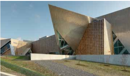
The Robinia wood façade of the Westside Shopping and Leisure Center in Bern-Brünnen, Switzerland artfully integrates into the surrounding rural countryside to the west.
