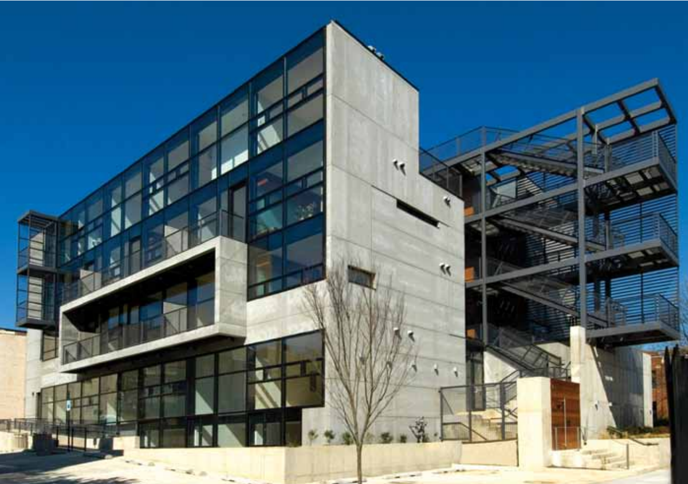
The industrial elegance of The Lacey's back elevation is Honarkar's favorite view of the building.
