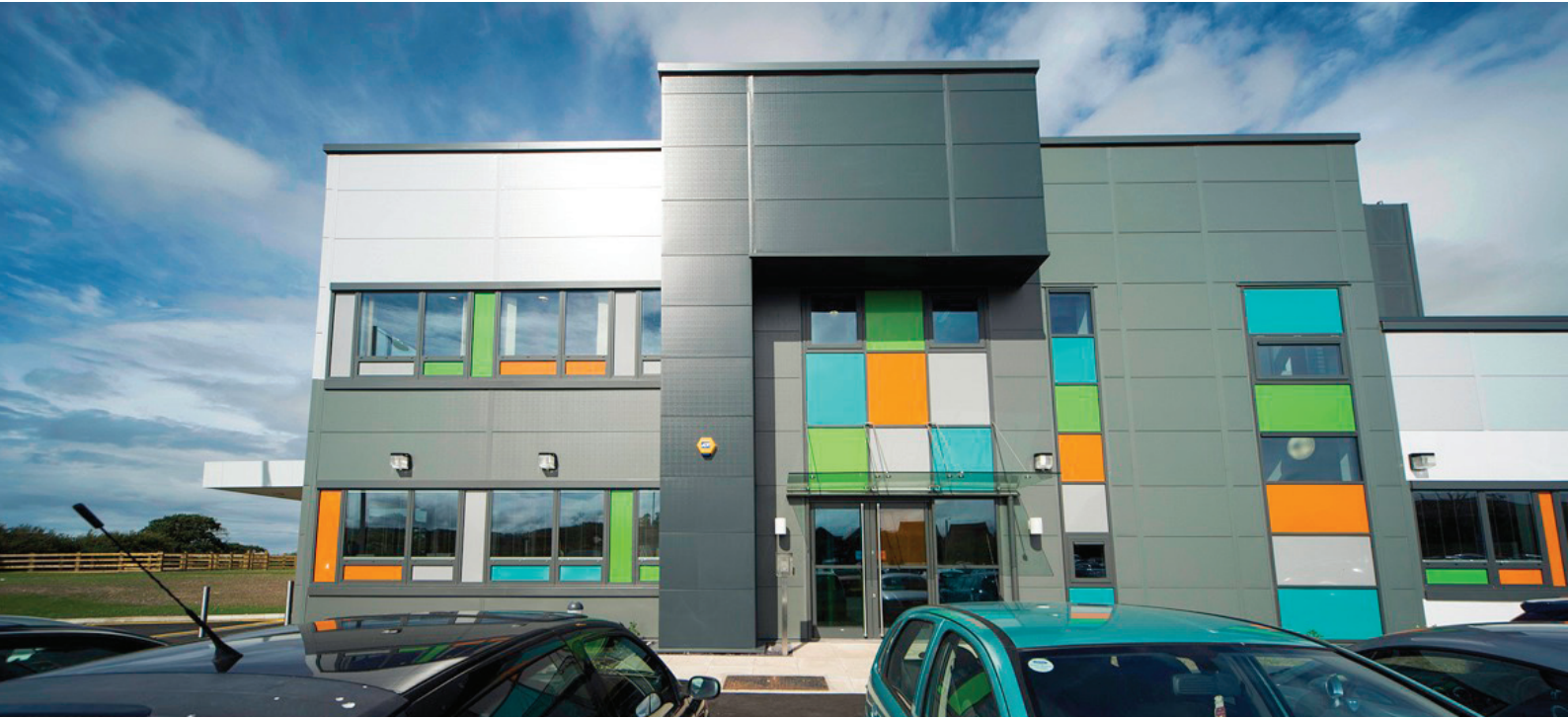
The Pathology Department building for the Ysbyty Glan Clywd Hospital was The Design Büro's first, large-scale BIM project.
