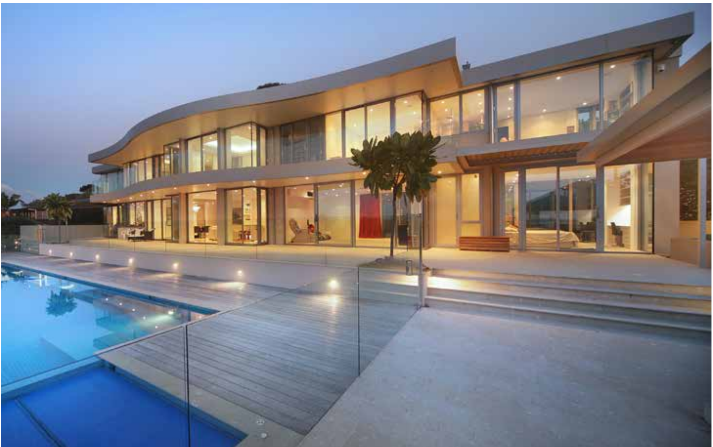
Farm Cove's living room, kitchen, theatre, and guest bedroom open to a large tiled outdoor terrace and infinity pool. The pool and hot water are on an energy-saving, passive-heating system.
