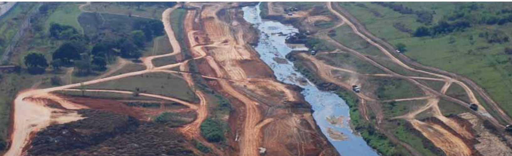
The Jacuba River drainage basin undergoes construction to make way for the revitalization project.
