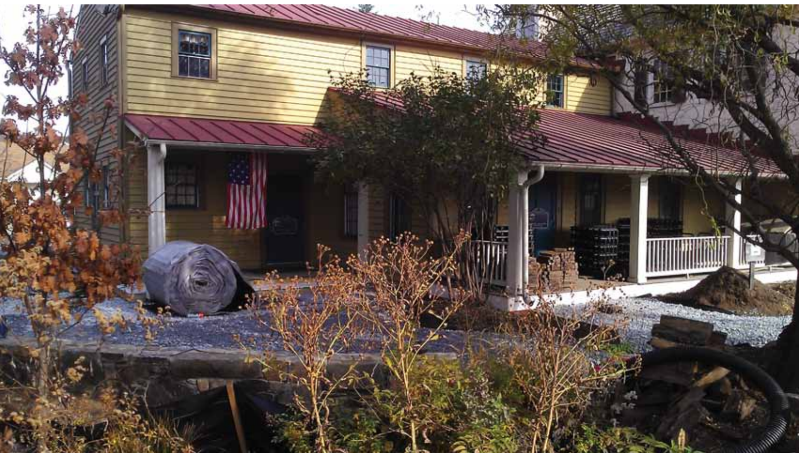
Designed to manage stormwater and runoff, the new cistern and other drainage solutions will reside primarily on the grounds in front of this portion of AWS' headquarters, located behind the original house.
