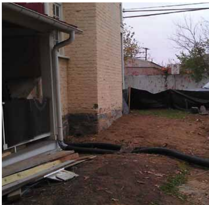
Work is in progress to prepare the site for the cistern and drainage solutions.
