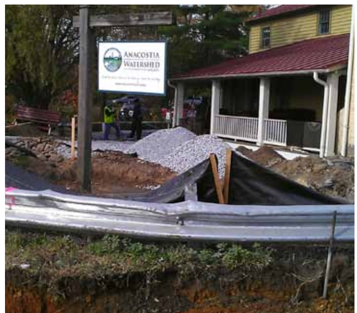
The house currently sits at an elevation below the road due to years of horizontal and vertical road realignments. Addressing the resulting negative drainage problem is central to this and future projects. The photos show before and in-progress views.
