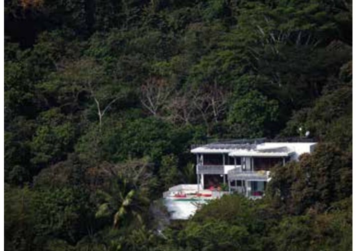
Located on a rain-forested mountainside in Costa Rica, the Casa Torcida house is 100% off the grid and is self-sufficient in its use of power and water.
