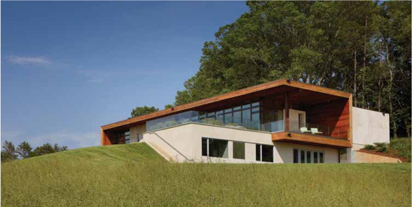
In the Asheville Leicester House, natural ventilation and large overhangs mitigate solar gain.
