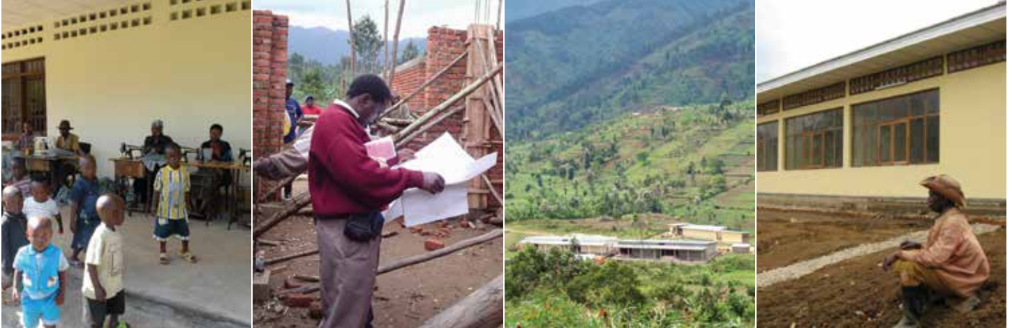
Local materials such as brick, stucco, and corrugated metal roofs are the primary building components at Kageno. The complex provides villagers with a place to commune, cook, learn, work, and access health care.
