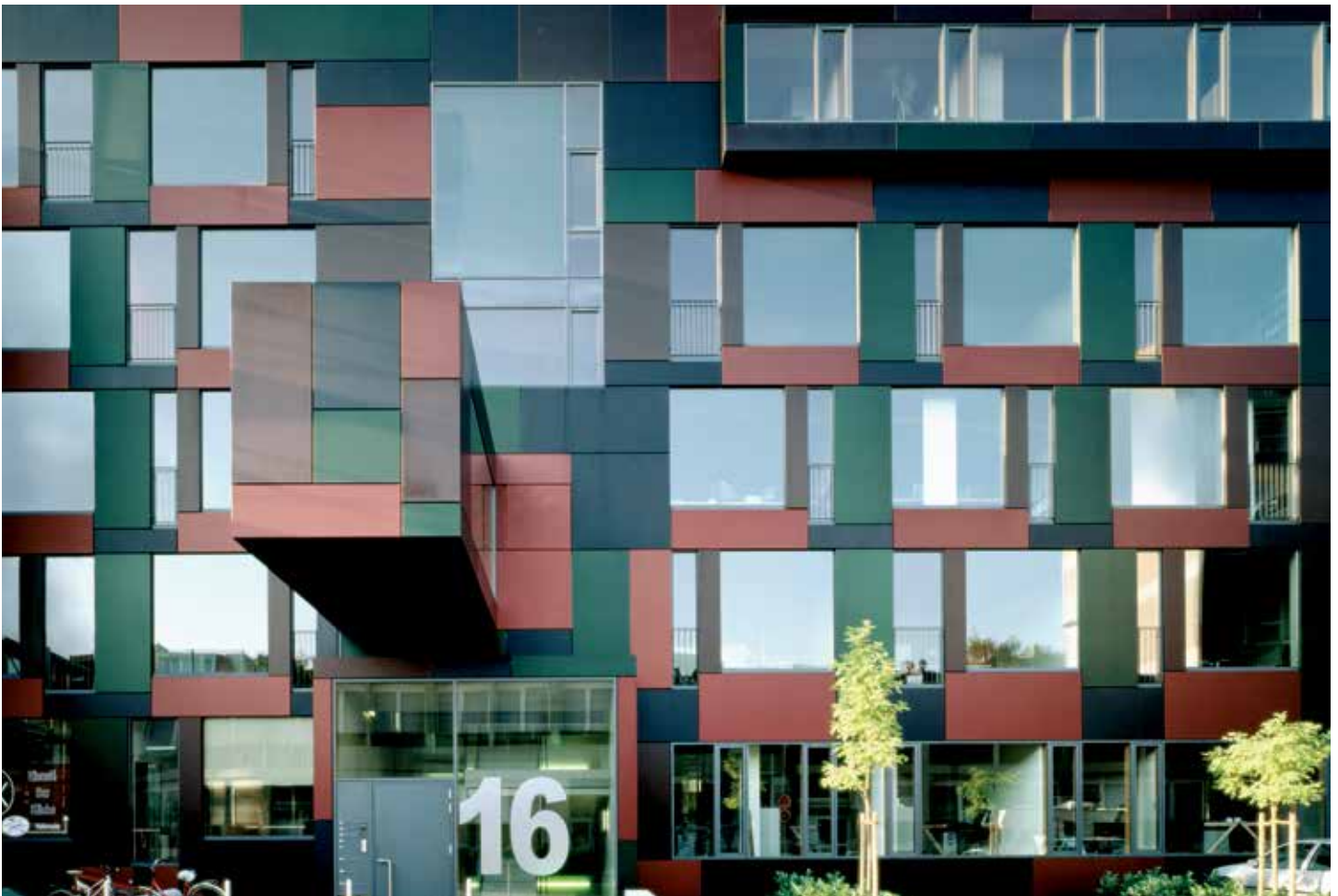
The office of BOLLES+WILSON features a colorful, anodized metal façade. Photo © Rainer Mader.
