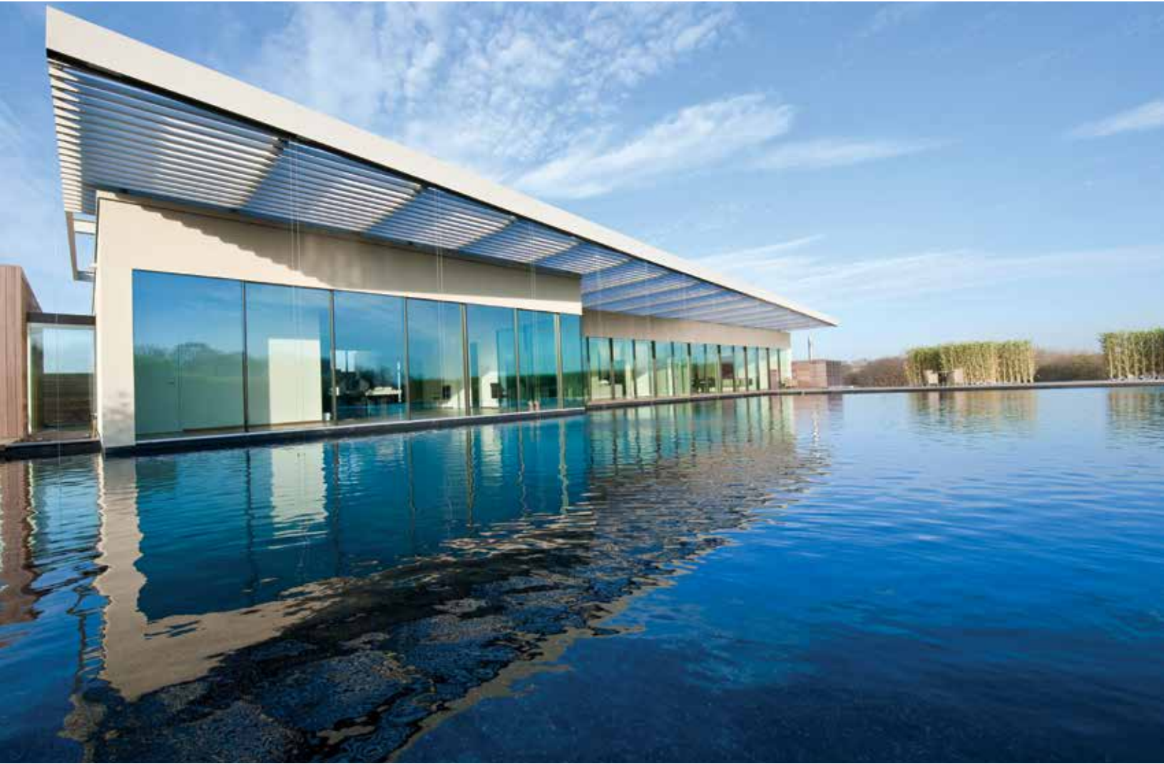
Visitors to the upper floors of the RS+Yellow building experience an element of surprise upon discovering a beautiful lake on the rooftop. Photo © Markus Hauschild, www.hauschild.biz .
