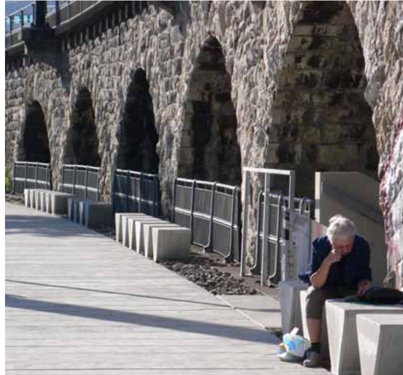
Above Left: A "before" look at the old viaduct prior to its redesign. Above Right: Concrete benches placed along The Lettenviadukt's new promenade function as logical resting places for walkers.
